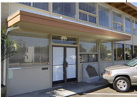
844 East Charleston Road, Palo Alto (2006). Photo by Dicklyon.
